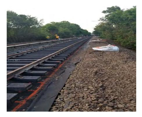
The photo depicts new trackwork, including new railroad ties, contact rail and running rail, that was recently replaced as part of Phase 1 of the Mainline Track Replacement Program along the Staten Island Railway in 4 sections between Huguenot and Clifton Stations that was part of Contract T-80280.
