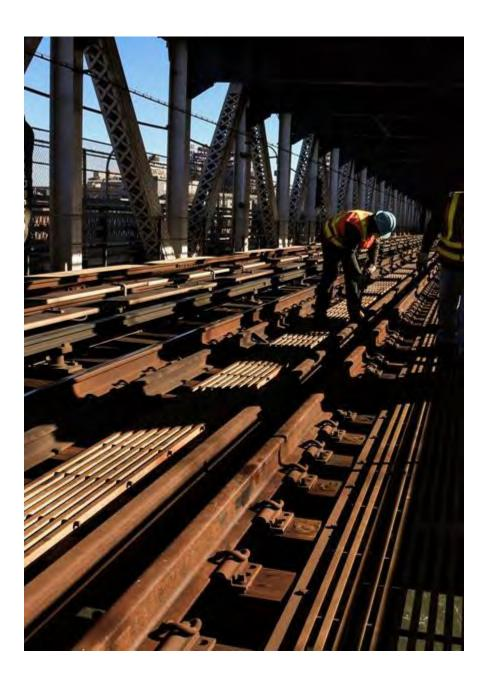
The New York City Subway has over 665 miles of mainline track, including almost 250 miles above ground on embankments, open cuts, elevated structures, and bridges. Here, team members perform important track maintenance high above the East River on the tracks used by the B and D Lines on the Manhattan Bridge.
