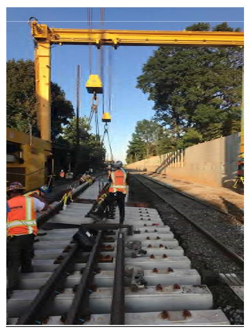
**Main Line Expansion**: As part of the ongoing project work, a new switch was installed within Nassau Interlocking on September 26, 2020.
