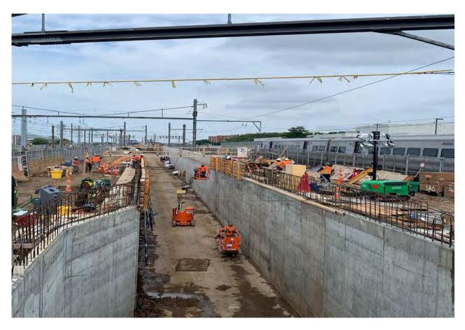
The picture above depicts the installation of formwork panels for the parapet walls in Harold Interlocking in Queens as part of the East Side Access Project. Harold Interlocking is the busiest rail interlocking in the Country. This month's agenda includes two procurement actions related to work in Harold Interlocking.
