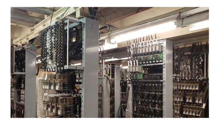
The above photo depicts the 36th St. Relay Room which was constructed as part of the Communications-Based Train Control System contract for the Queens Boulevard Line. This equipment is utilized to monitor and control the switches and signal equipment of the 36th Street interlocking portion of the Queens Boulevard Line.
