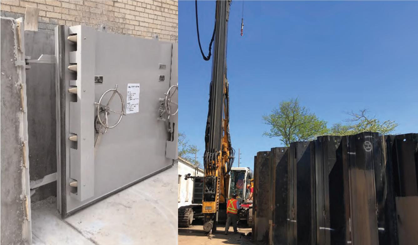
FIGURE 6: DUAL PURPOSE FLOOD AND DEBRIS WALL INSTALLED AROUND HAMMELS WYE FACILITY AND FAR ROCKAWAY BRANCH.
