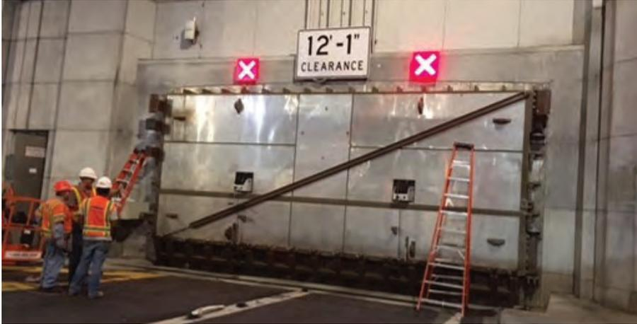
FIGURE 13: PORTAL FLOOD GATE AT HLCT MANHATTAN WEST IN CLOSED POSITION
