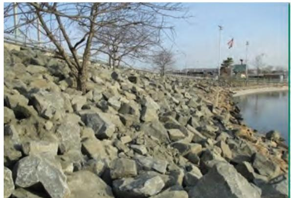
FIGURE 17: RESTORED ABUTMENT AT CROSS BAY BRIDGE
