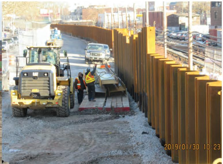
FIGURE 5: INSTALLATION OF THE PERMANENT PERIMETER FLOOD BARRIER AT CONEY ISLAND YARD.
