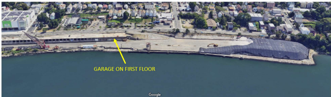
Figure 4: The western half of the Atlantic terminal. The garage occupies a long section of the tunnel. The removal of the upper stories of the 840-foot-long building removed some hazards while creating an opportunity for views from a BRT at street level.
