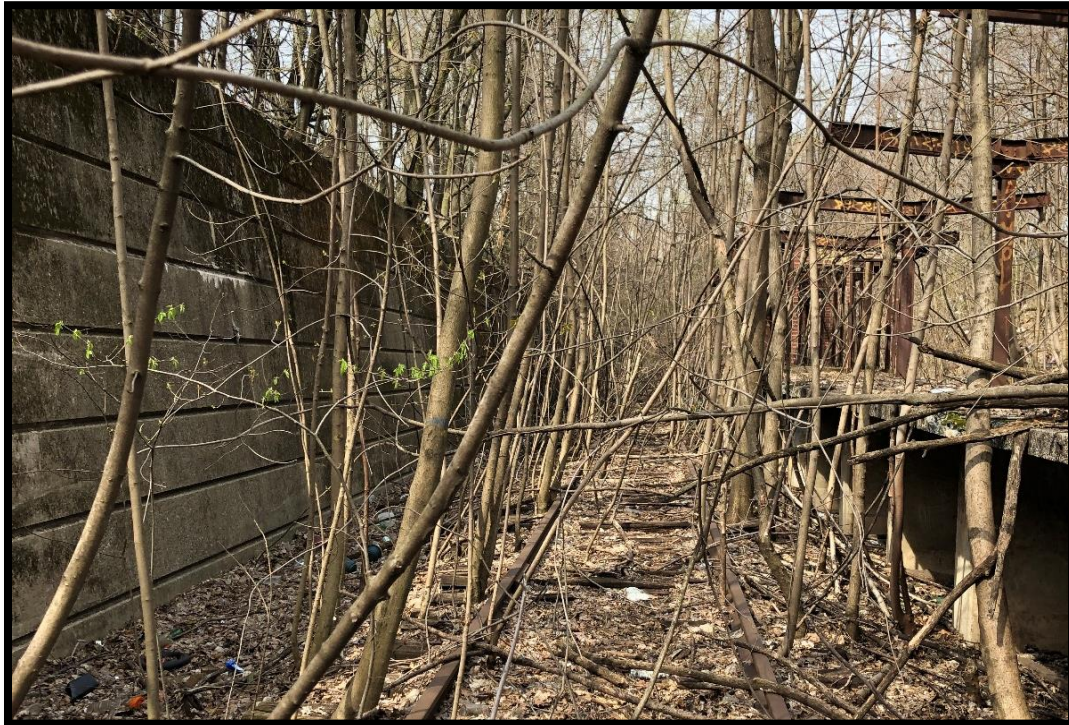
Photo N: View looking west at early successional vegetation along the abandoned rail line near the old Mariners Harbor station platforms. Early successional communities dominated by exotic species are common along the rail portion of the entire study area.
