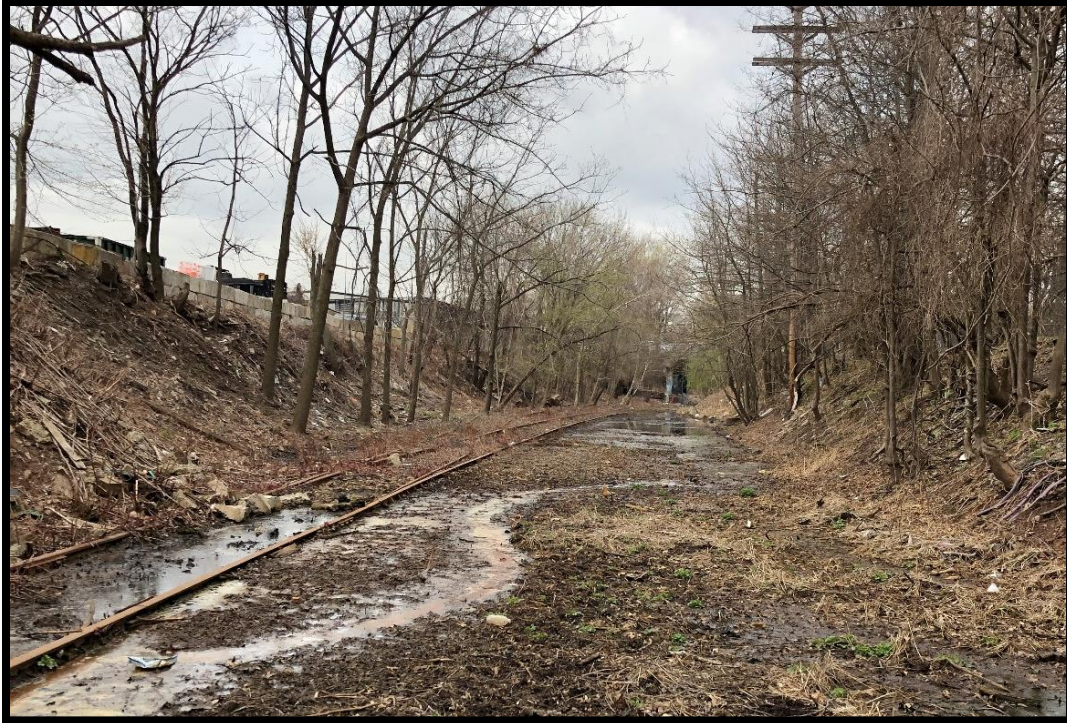
Photo Q: View looking west at the recessed train line just west of the Bayonne Bridge. Ponded water was common within the recessed portions of the line, however these areas consistently lacked hydric soils and/or were underlain with gravel ballast.
