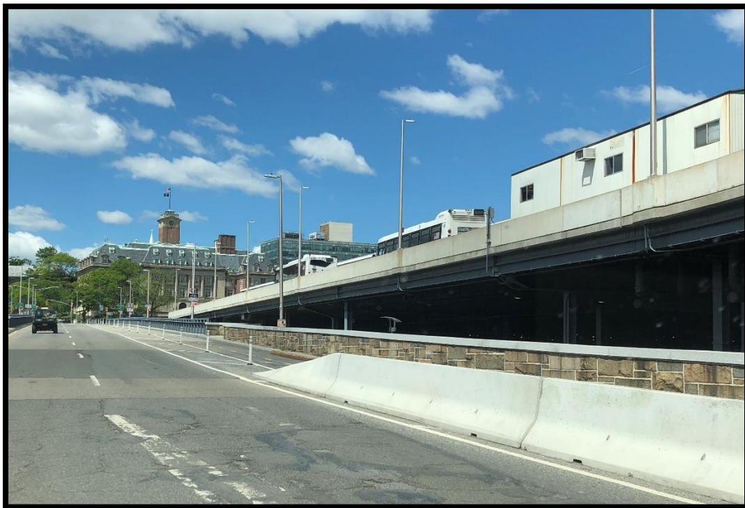
Photo HH: View looking south from the Staten Island Ferry Viaduct at the eastern end of the study area.
