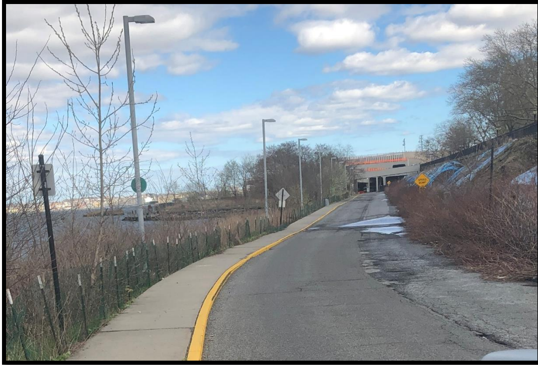
Photo GG: View looking east along the parking garage access road (north of Richmond Terrace) showing mid-successional upland growth and bulkhead along the shoreline.
