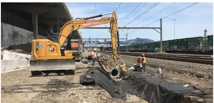
PSA construction workers install drainage system near Leggett Interlocking
